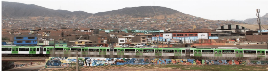
View of Line 1 Metro Lima
